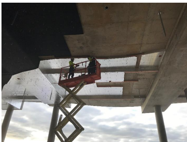
Rigid soffit insulation being installed
